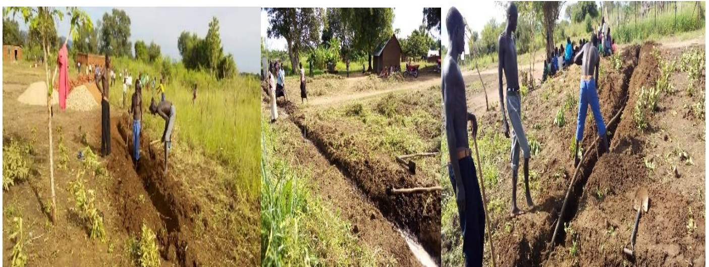
Channel digging for Water yard extension pipe during rehabilitation of water distribution systems in Enyif village and Enyif primary school.
